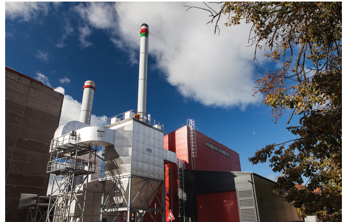
Liepaja biomass facility
